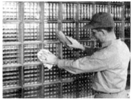
FIGURE 11.15 (Top left) First step in installation of a glass-block panel is to coat the sill with an asphalt emulsion to allow for movement due to temperature changes. Continuous expansion strips are installed at side and head jambs. (Top right) Blocks are set with full mortar joints. (Bottom left) Welded-wire ties are embedded in the mortar to reinforce the panel. (Bottom right) After all the blocks are placed, joints tooled to a smooth, concave finish, and the edges of the panel calked, the blocks are cleaned.
