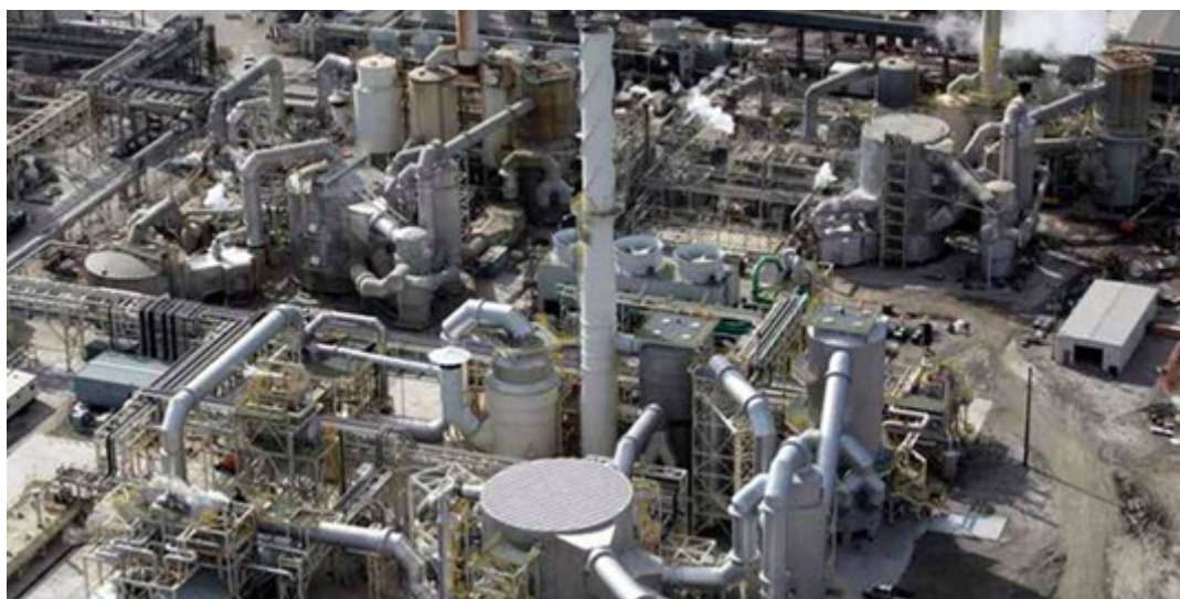
Sulfuric acid plant [DSD Chemtech]
