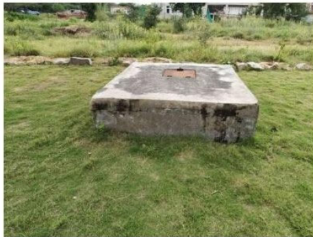
Water harvesting chambers in the college premises
